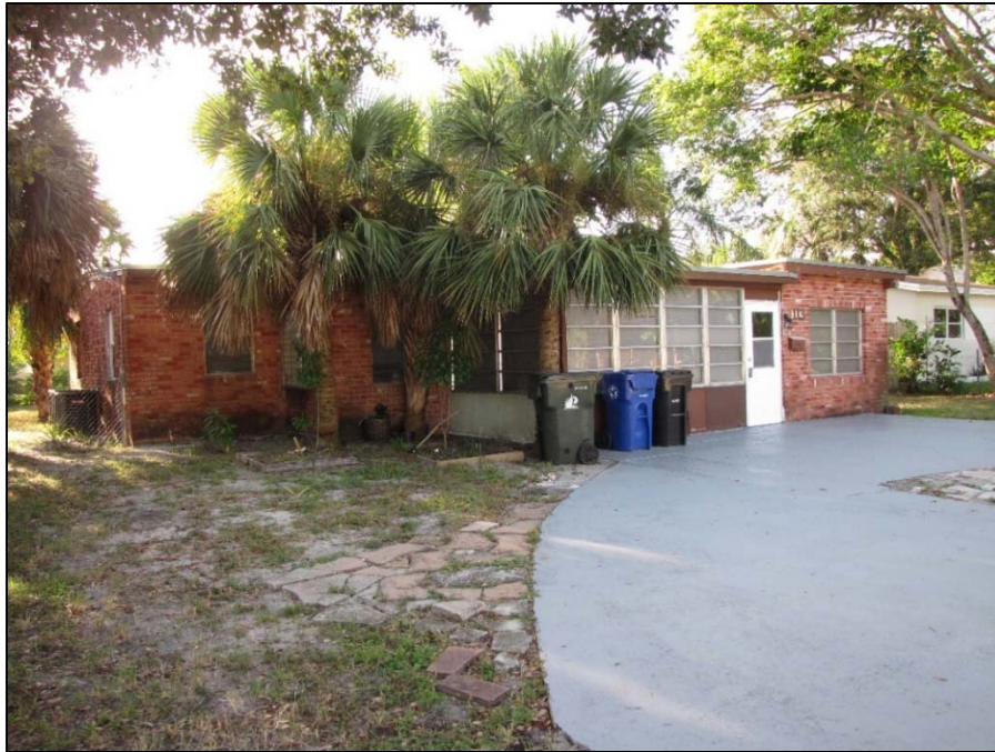
Figure 39 | 109 SW 21 st Way (8BD6777), c. 1953, facing West, exhibits enclosed carport and porch, replaced windows and doors, northeast corner addition
