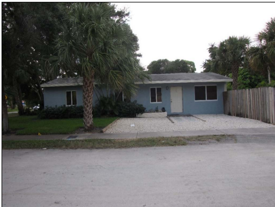
Figure 13 | 23 SW 22 nd Avenue (8BD6751), c. 1952, facing West exhibits enclosed carport, replaced windows and doors, and northwest corner addition
