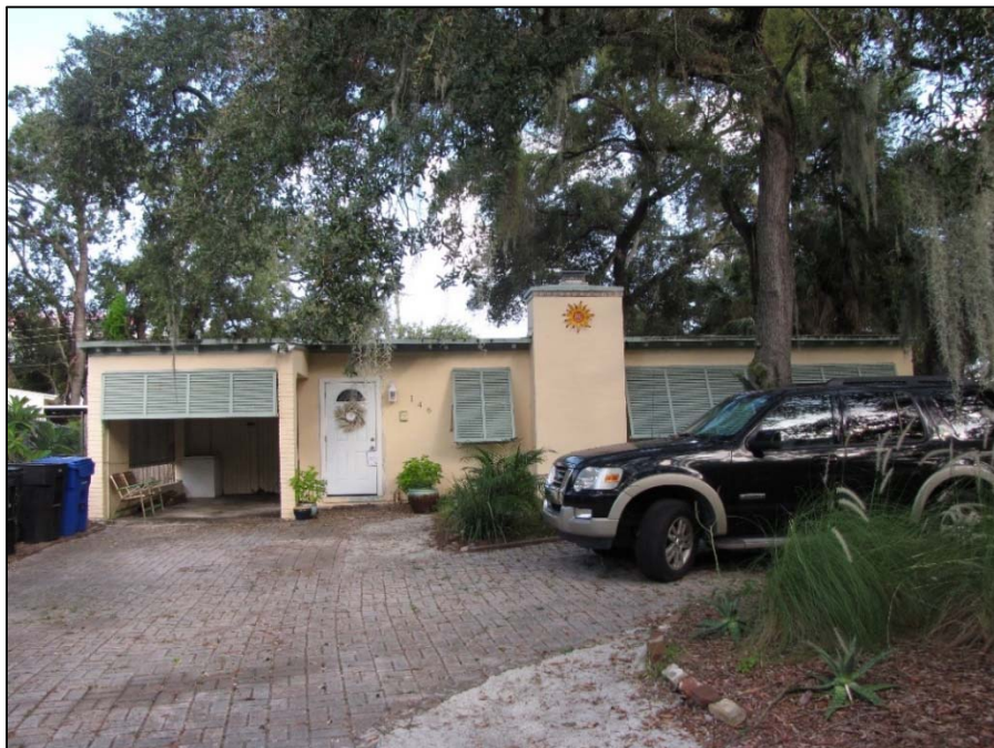
Figure 30 | 200 SW 21 st Way (8BD6768), c. 1953, facing Northeast, exhibits enclosed carport, screened in porch, replaced windows and doors, northeast corner addition
