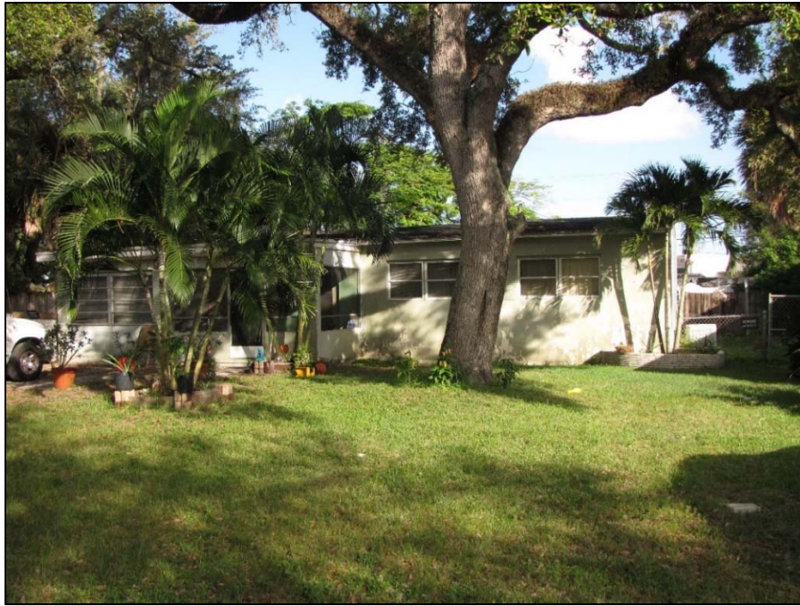
Figure 31 | 204 SW 21 st Way (8BD6769), c. 1953, facing South, exhibits enclosed porch, replaced windows and doors, northwest and southwest corner additions
