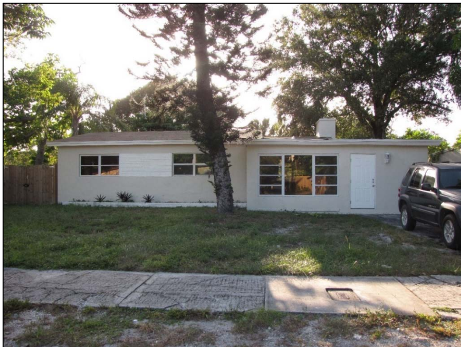
Figure 40 | 105 SW 21 st Way (8BD6778), c. 1953, facing West, exhibits enclosed porch, replaced windows and doors
