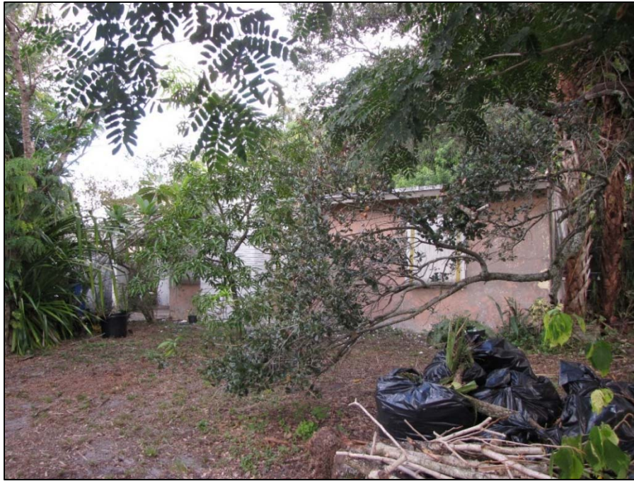
Figure 27 | 138 SW 21 st Way (8BD6765), c. 1953, facing Northeast, exhibits enclosed porch, replaced windows and doors, northwest corner addition
