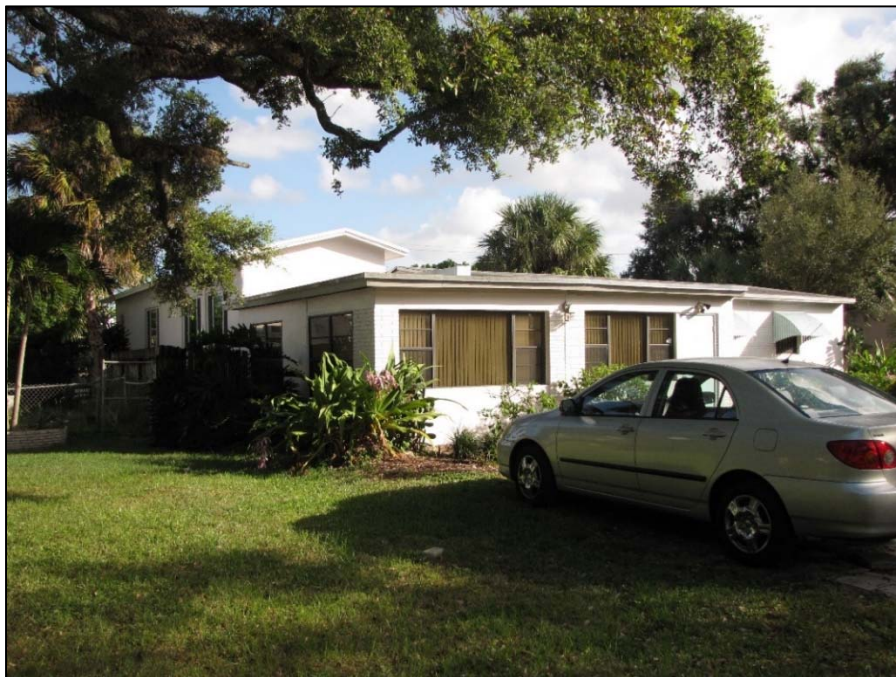
Figure 32 | 143 SW 21 st Way (8BD6770), c. 1953, facing Northwest, exhibits enclosed porch, replaced windows and doors
