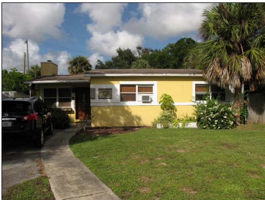
Figure 18 | 2121 SW 1 st Court (8BD6756), c. 1953, facing East, exhibits replaced windows and doors, northwest corner addition
