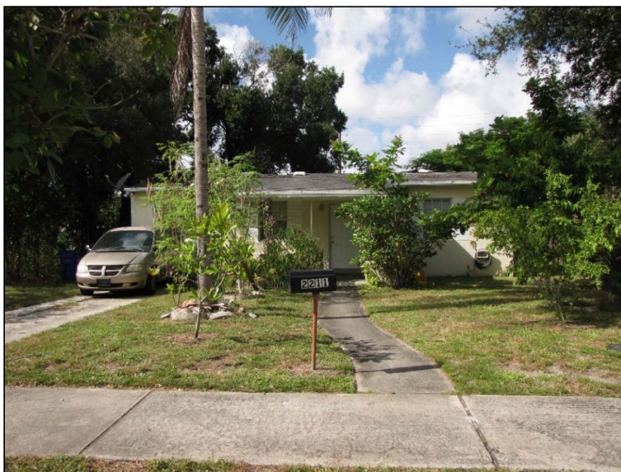
Figure 11 | 2211 SW 1 st Court (8BD6749), c. 1953, facing North, exhibits enclosed carport, replaced windows and doors, and a north side addition
