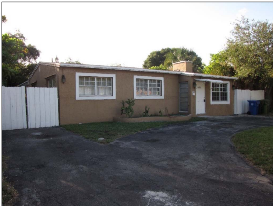
Figure 38 | 113 SW 21 st Way (8BD6776), c. 1953, facing Northwest, exhibits enclosed carport and porch, replaced windows and doors
