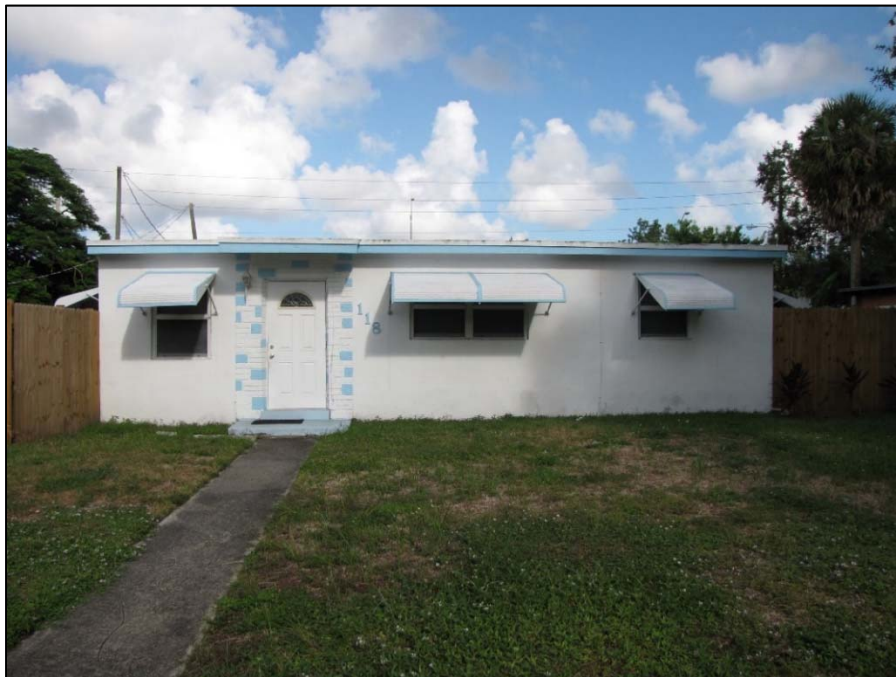
Figure 24 | 124 SW 21 st Way (8BD6762), c. 1953, facing East, exhibits enclosed carport, replaced windows and doors
